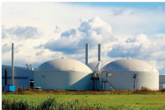
Methane produced by digesters is sold to biogas companies that convert it to electricity.
